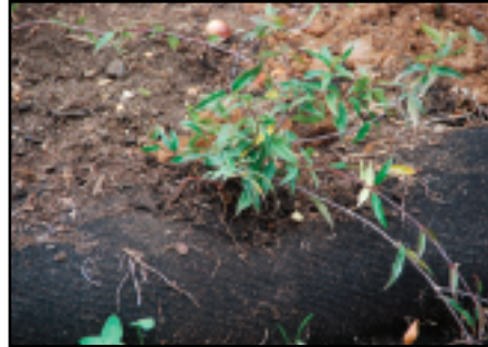
Compost socks can be planted with live stakes or plugs at installation.
