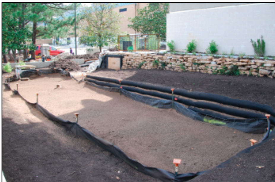
Bioretention system at Southface using compost socks, compost engineered soil, and compost blankets.
