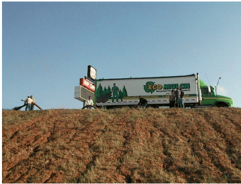
Rills are often obvious on steep or unprotected banks.
