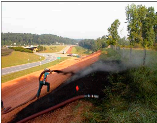
Figure 2 Slope application of compost blanket
