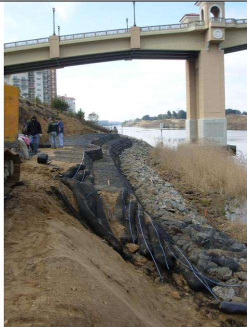
Sock wall locked in place with geotextile
