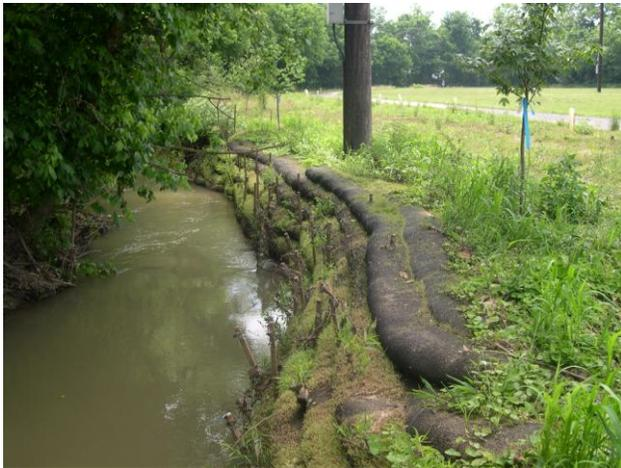
Compost filter sock used in stream bank stabilization
