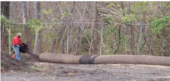
Figure 7. Installing a 24" Filtrex SiltSox. Photo by Cary Oshins
